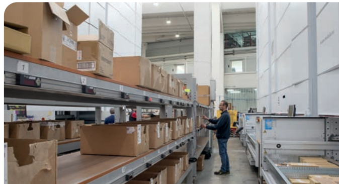
Put-to-Light systems connected to WMS
